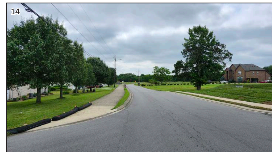
View of From Biraj Court & Tway Court Intersection Looking Southeast
