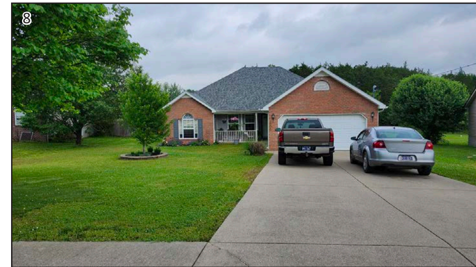
View of Neighboring Residential Home Looking North
